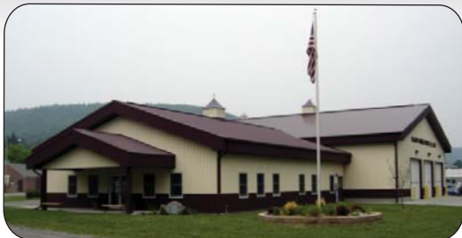
Grand Gorge Fire Station Project
