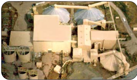
Aerial Photo of Simplot Phosphates, LLC facility located in Vernal, Utah.
